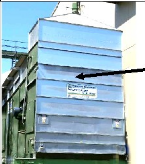
Models from 1000 to 2200 bu/hr. DF22 19'H high end, 14' wide, 40' long, 12' H @ low end
